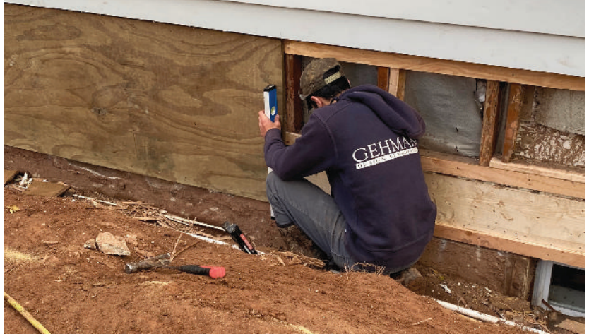
Gehman's team installs pressure-treated sheathing as part of its solution to fix the damage.
