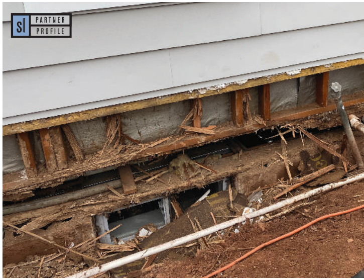
Water caused significant damage to the home of this Gehman Design Remodeling client in Harleysville.
